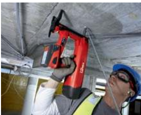
Threaded rod attachments to concrete
