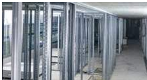
Drywall tracks to concrete and steel
