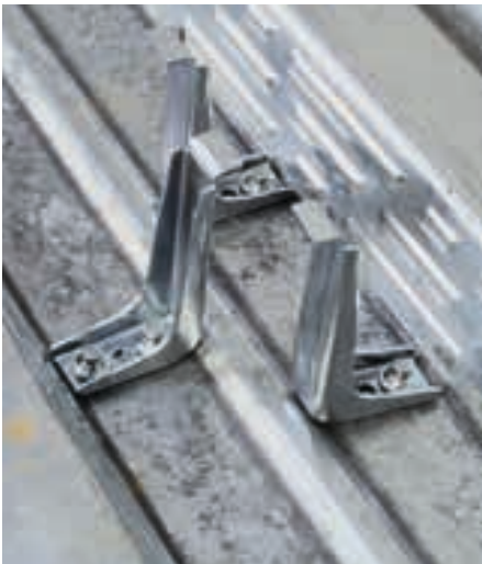
Figure 6: Hilti X-HVB installed on profiled deck
