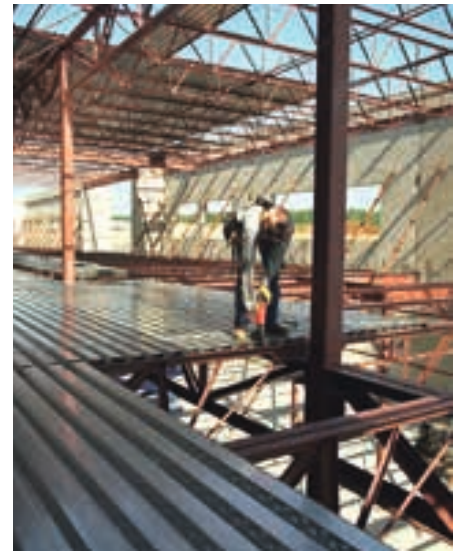
Figure 1: Installation of profiled sheeting for a composite slab
