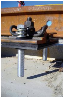
Clipped components before concrete pouring
