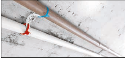
X-UCT-E MX with cable ties for two pipes
