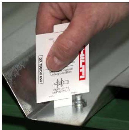
Checking the standoff of an ENP2 roof deck fastening with a plastic gauge
